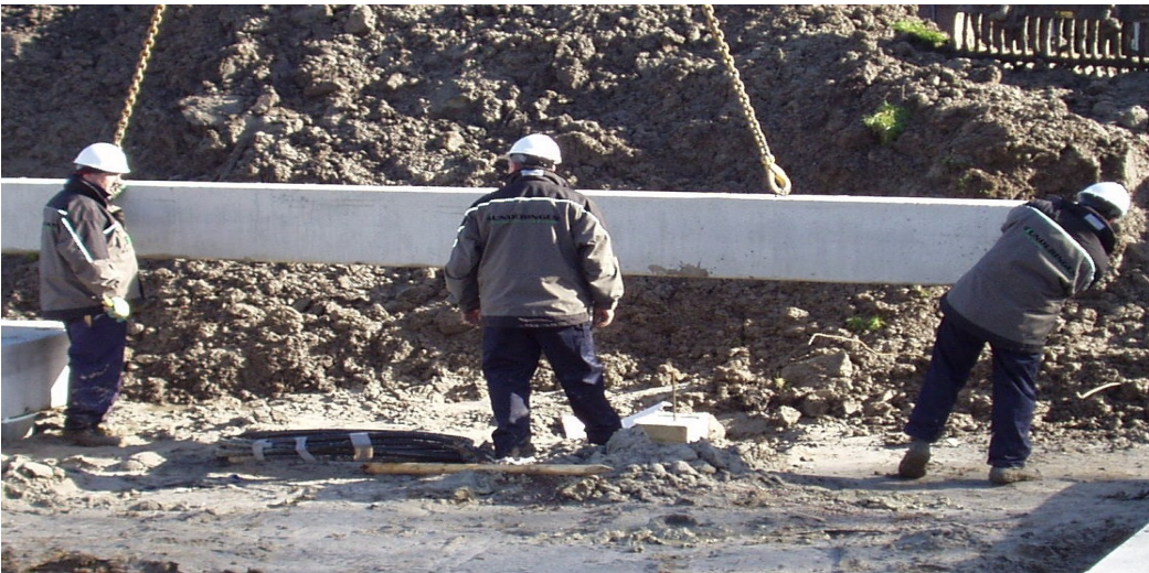
Montage prefab heifundering
